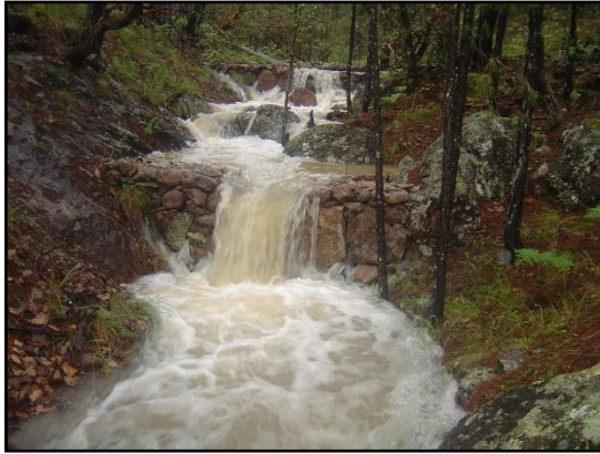
Figure 9. Thousands of gabion and check dam structures have been installed along upper tributaries of the Rio Conchos to slow runoff, capture sediment and encourage ground water recharge (photo by Alfredo Rodriguez, WWF).
