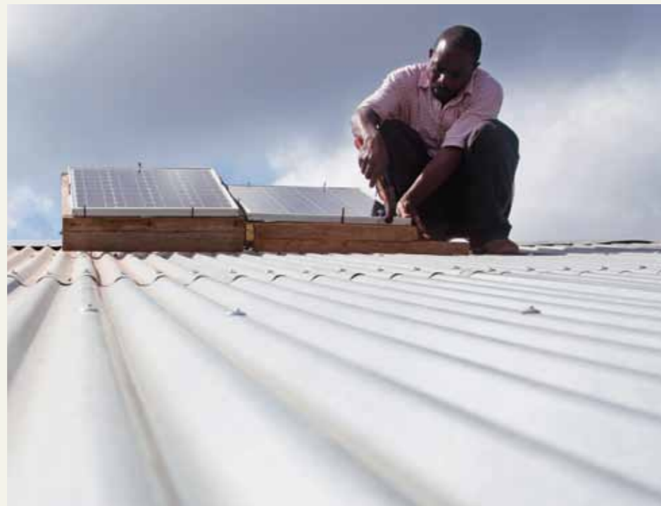
Technician fitting solar panel on a corrugated iron rooftop, Miono region, Tanzania, Africa.
