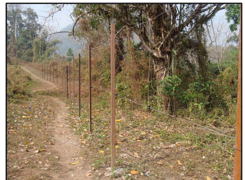
4.5 km solar fencing
