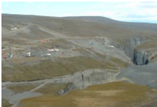
Construction site for the Kárahnjúkar dam in the East Icelandic highlands
