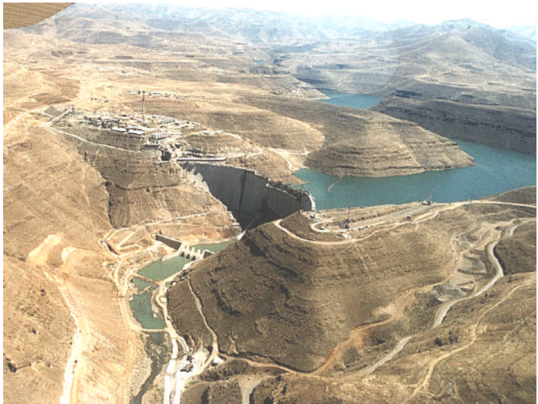
Figure 14: The 186 m. high Katse dam (Africa's highest) under construction © Martin Rigby
