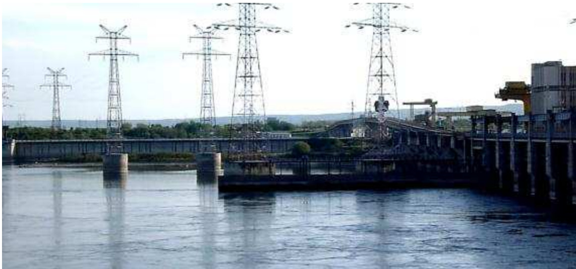
Fig. 18 View from left bank on the tailrace of the Serbian side of the dam (picture O. Calles)
