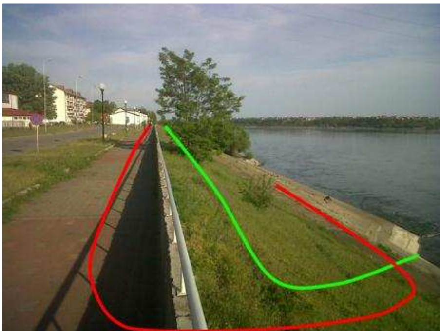
Fig. 25 Two possible paths of the downstream section of the bypass channel – F.P. A (picture O. Calles)
