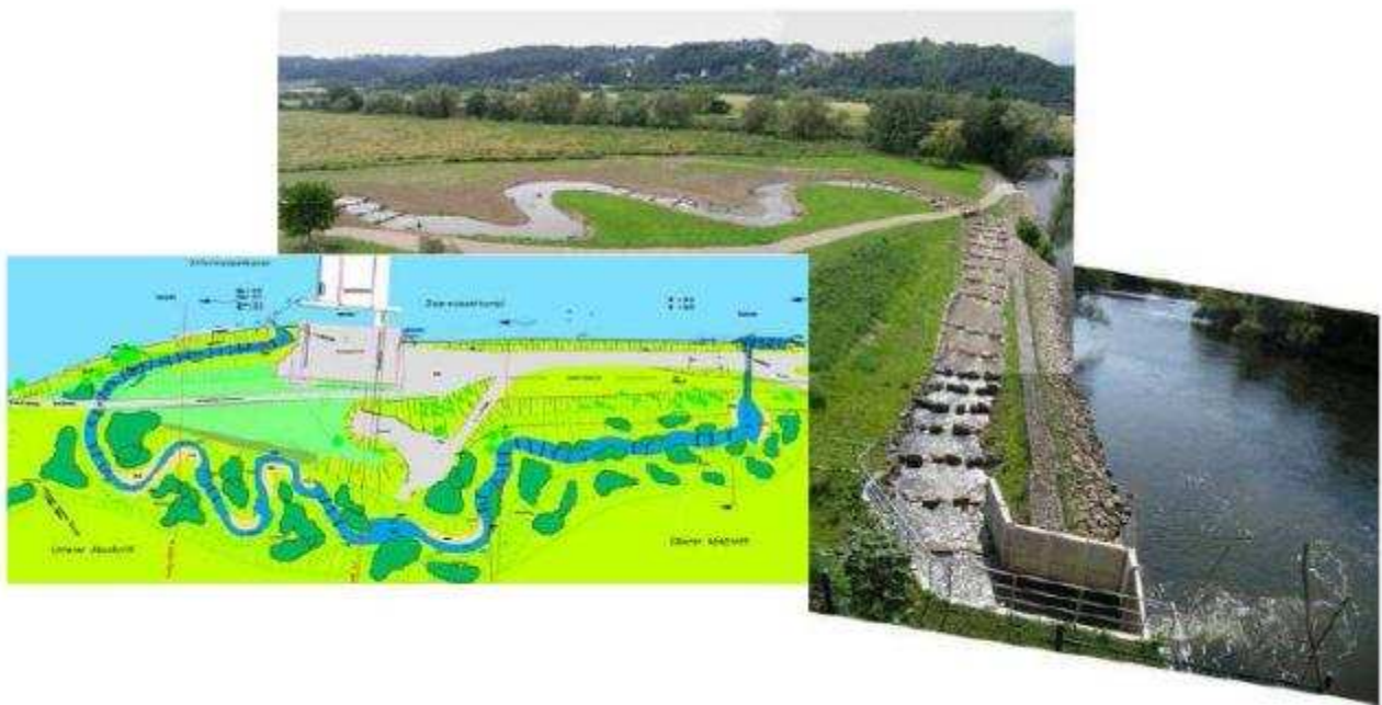
Fig. 27 Bypass channel at Harkort dam on river Ruhr, Germany (from Gebler, 2007)
