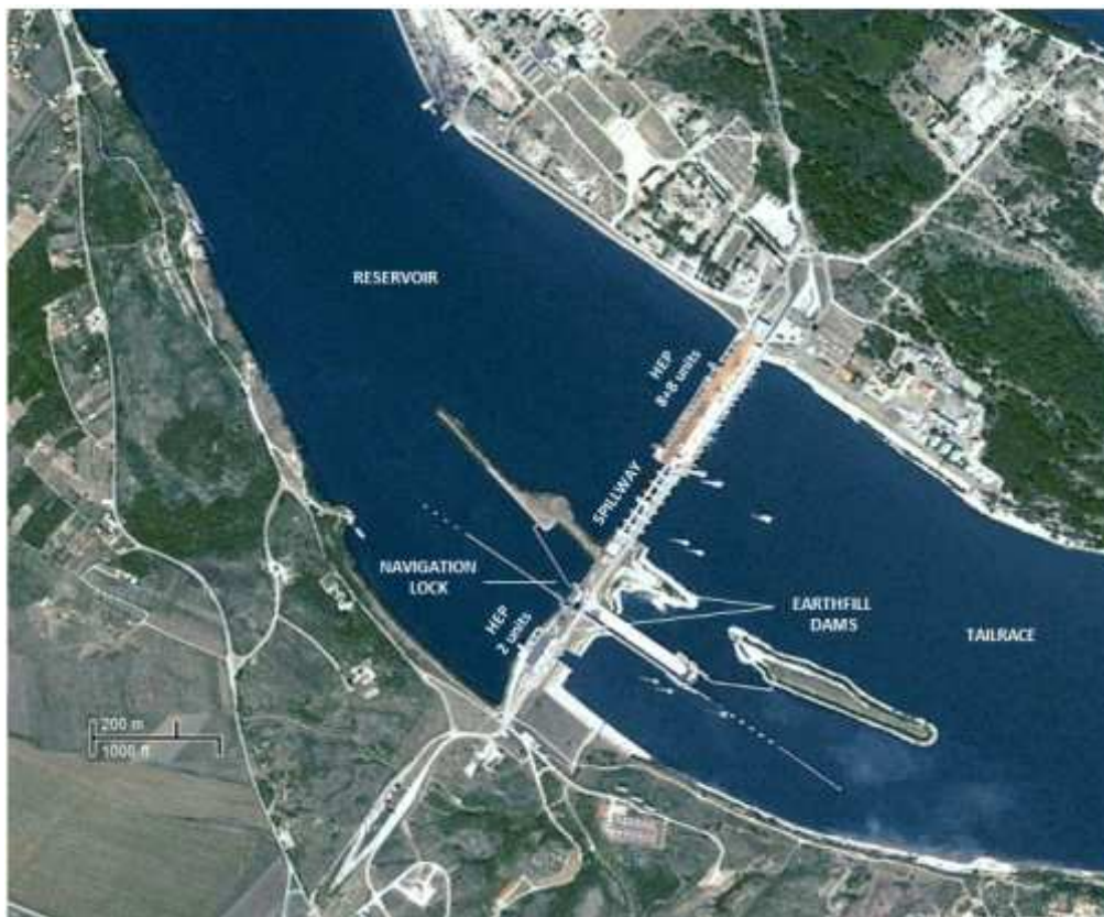
Fig. 16 Iron Gates II lower dam (from Google Maps)
