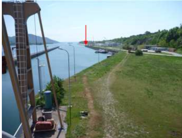
Fig. 40 Possible location of the bypass channel (F.P. F) entrance; on the left: navigation lock wall (picture O. Calles)
