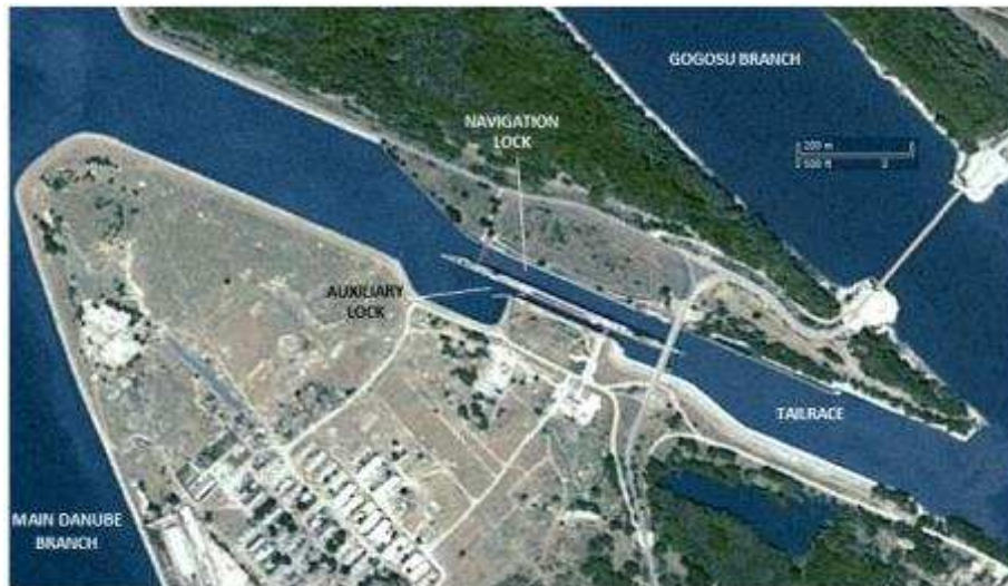
Fig. 13 Navigation locks through Ostrovul Mare island (from Google Maps)
