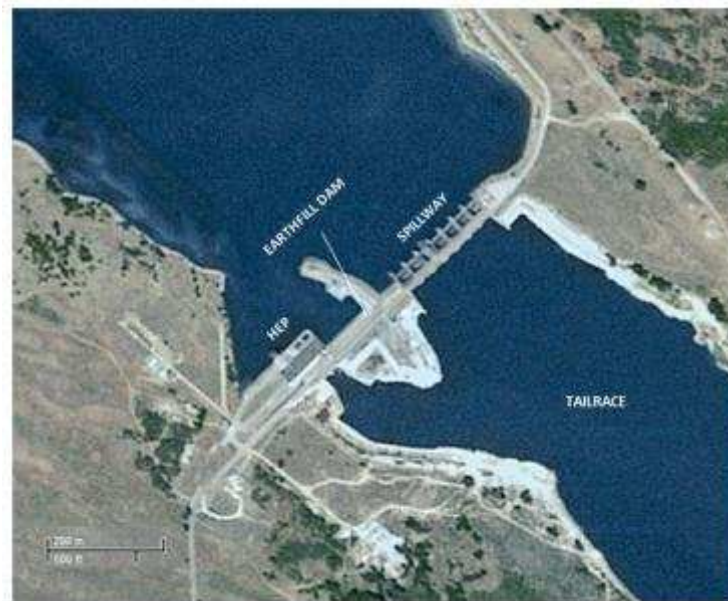
Fig. 11 Iron Gates II upper dam on Gogoşu branch (from Google Maps)
