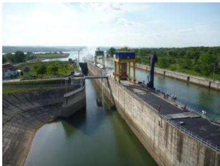
Fig. 14 View towards upstream on the auxiliary (left) and main (right) navigation lock (picture O. Calles)
