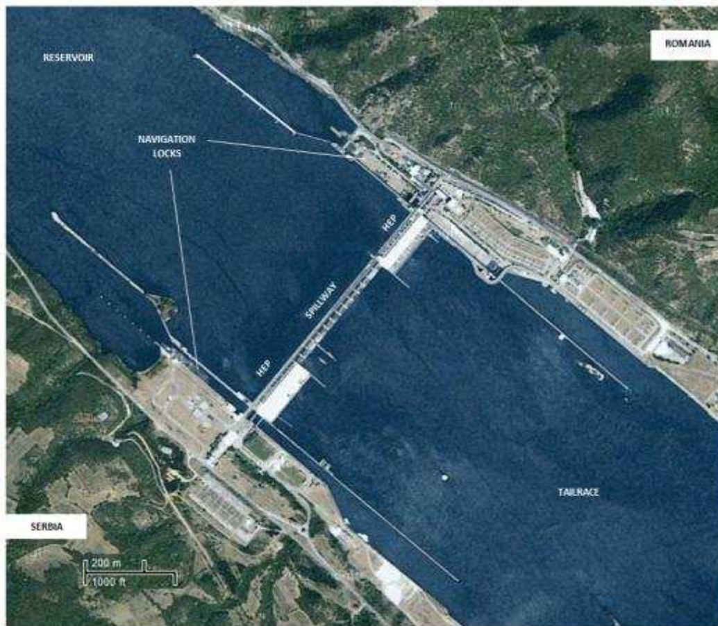
Fig. 4 Plan view of Iron Gates I dam (from Google Maps)
