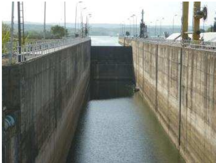
Fig. 36 View on the upstream sluice of the auxiliary navigation lock (picture G. Marmulla)
