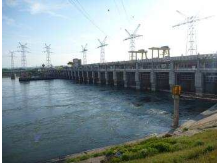
Fig. 17 View from left bank on the tailrace of the main HEP (picture O. Calles)
